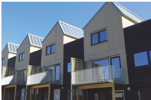
Terraced housing estate "Stenbråtlia" near Oslo. Thirty-four terraced houses, built to passive house standards, were equipped with roof-integrated polymer solar collectors from the company Aventa. This system meets 60 percent of the total energy consumption of both the hot water and the space heating. ©Aventa
