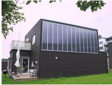
Fig. 2. Façade integrated polymeric collectors, passive house in Rudshagen, Oslo. (Source: Aventa)
